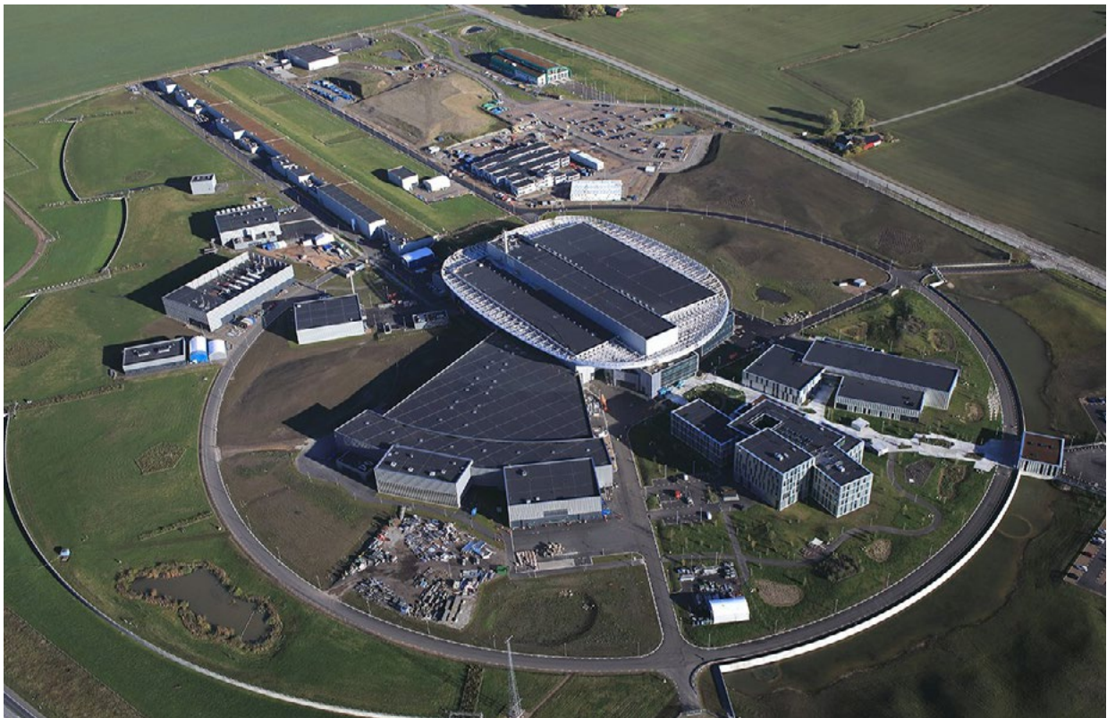
Aerial overview of ESS, European Spallation source. Photo: Perry Nordeng/ESS
